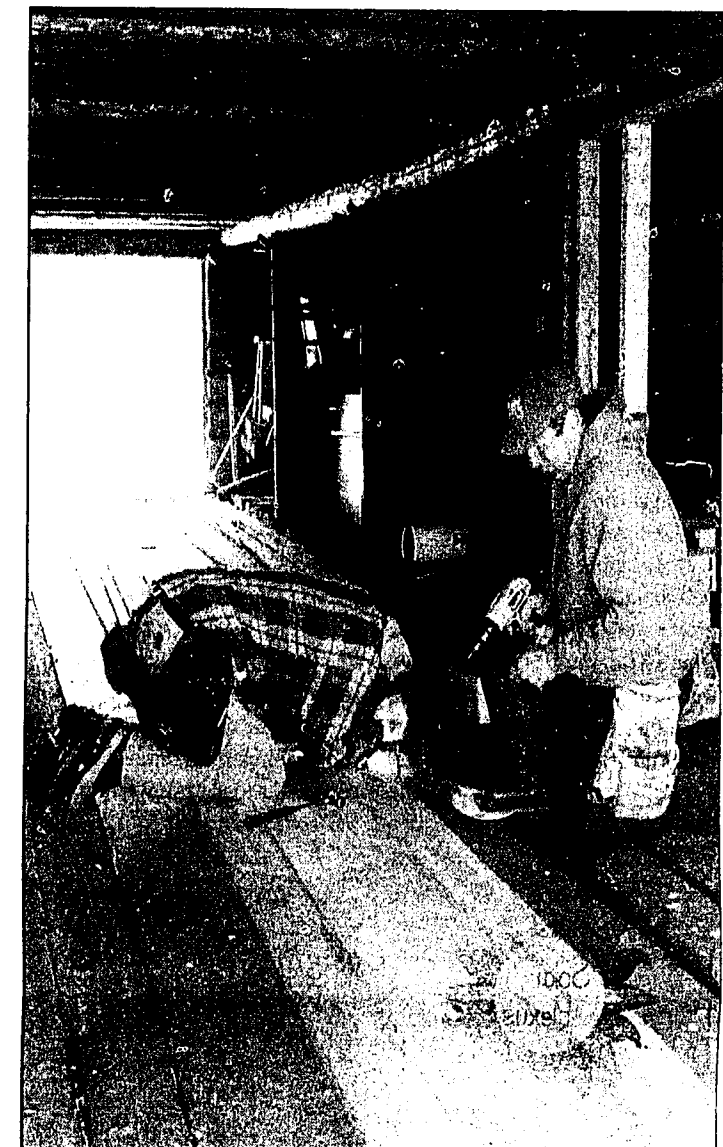
Shawn Ellinghouse and Bill O'Brien of Lake Country Builders work on the floor of the Seeley Lake Historical Museum and Visitor's Center. The last grant from the Historical Museum at Fort Missoula is enabling some construction to be done this spring.
