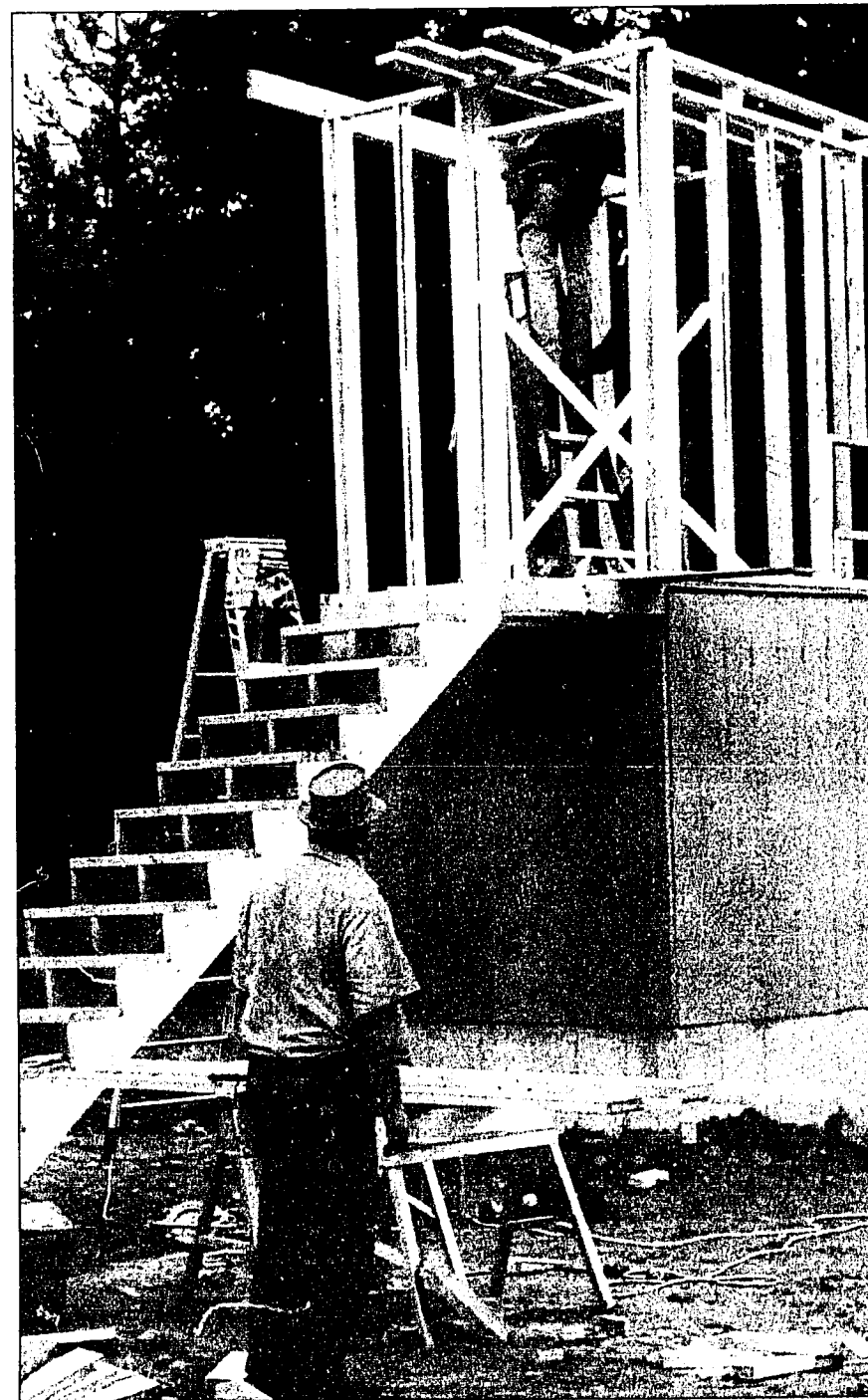
Work progressing on high skeet house.
