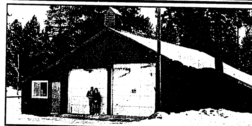
Duane Boulé, fire district manager, and Mary Marshall, fire district clerk, will soon be using office space located in the new addition to the Seeley Lake Firehouse. Volunteers also recently constructed a cold storage room (right).
